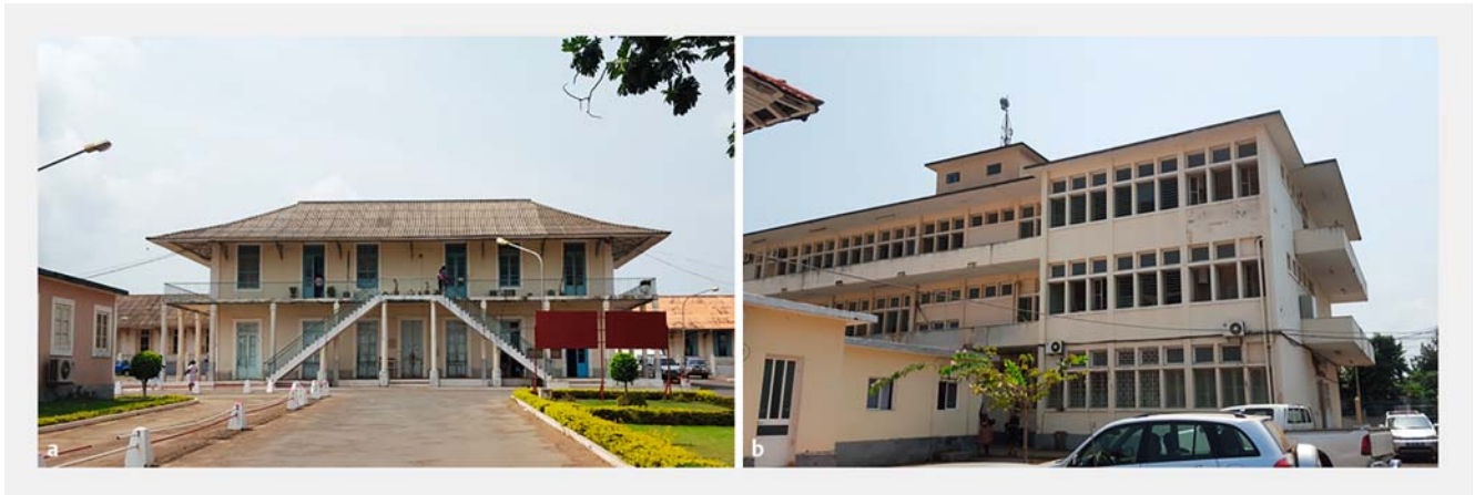
► Fig. 1 Dr. Ayes de Menezes Hospital, STP. a Main building. b Gastroenterology and General Surgery building, including endoscopy unit, Surgical Operating Room and Nursery.
