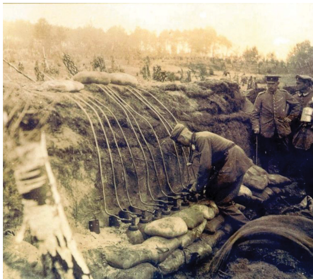
Figure 1. German battery of chlorine gas cylinders being prepared for an attack, awaiting the right weather conditions to prevent blowback; similar to the arrangement at Hill 60 in May 1915, open domain.
