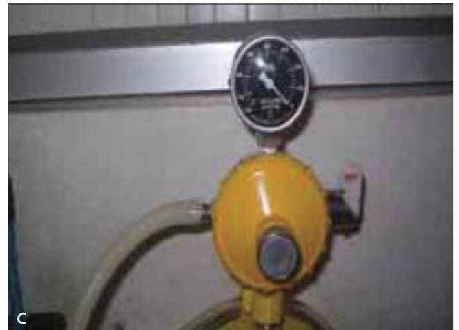
Figure 2c: Photograph showing the pressure gauge of the wall suction apparatus
